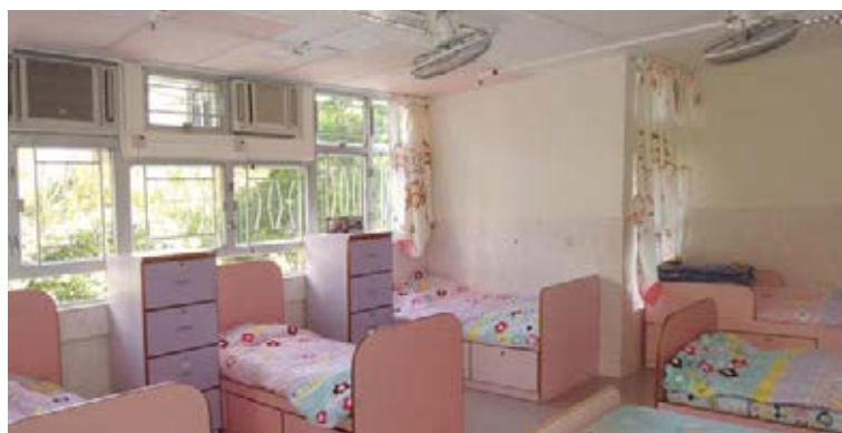
景林宿舍擴大房間窗戶面積，增加空氣流動及照明。 King Lam Hostel expands the window areas of rooms to increase air flow and improve lighting.
